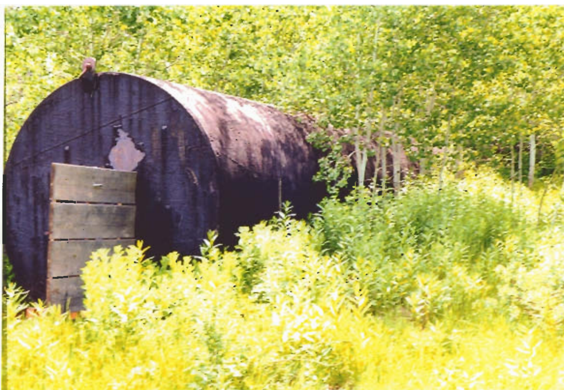
10 – View looking east at water supply tank and wooden valve box. Note that hasp is damaged and valve box cannot be locked.
