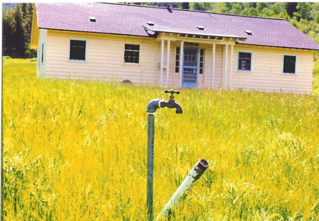
5 – View looking southeast at hose bib and two-inch galvanized pipe serving an unknown purpose. Note administration building in the background.
