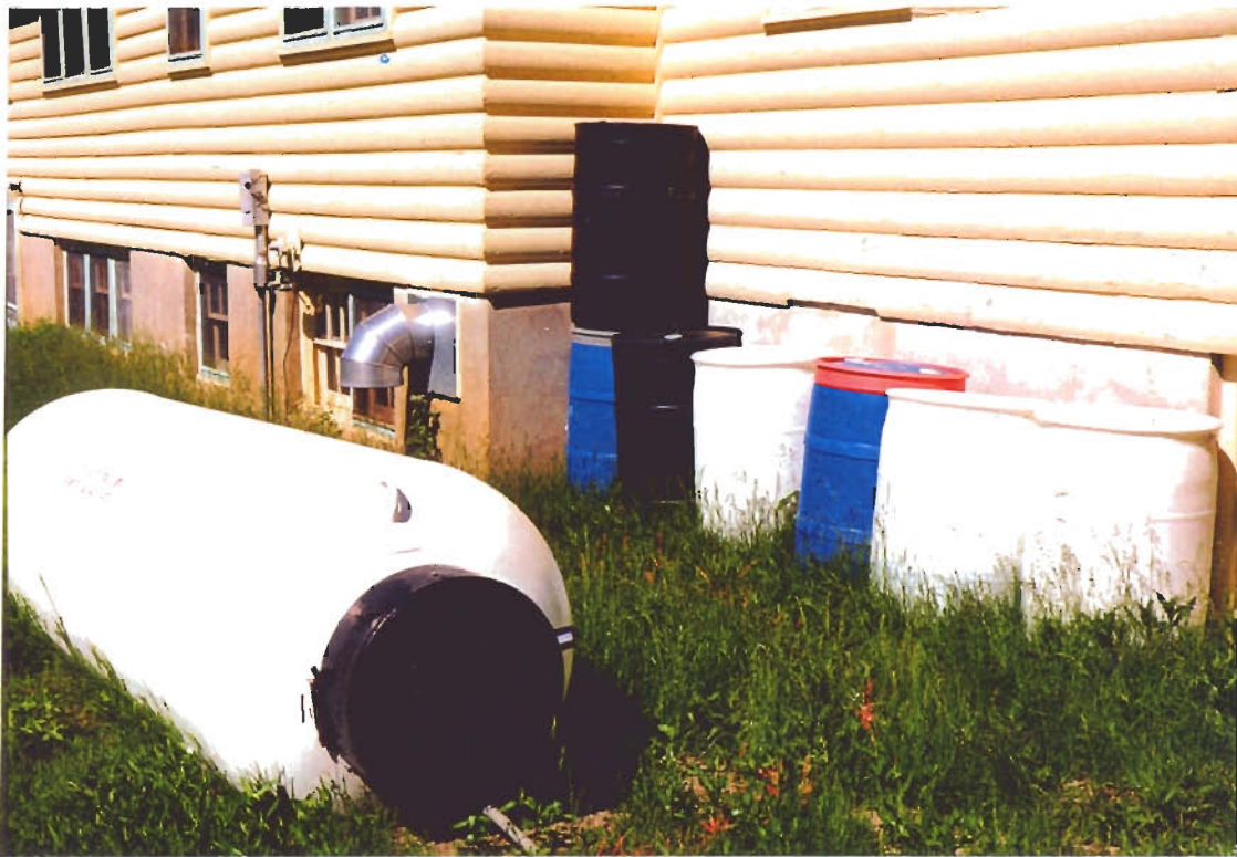
3 – View looking north at propane tank and seven plastic drums behind administration building.
