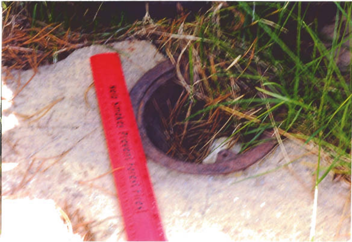
7 – View looking at open cast-iron drain or filler pipe located along western edge of the concrete pad for the propane tanks.
